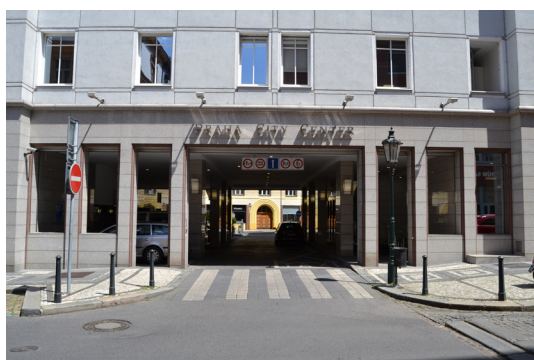
vstup z ulice Samcova / entrance from Samcova street
